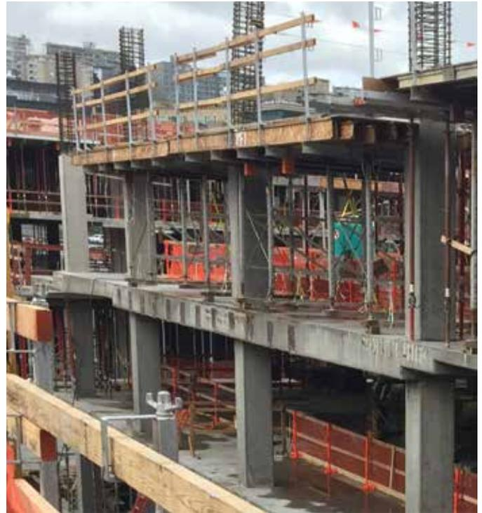
Because the SAPS guardrail system can be mounted inboard of the perimeter shoring towers, workers need to set the guardrails only once, prior to releasing and flying the exterior forms and towers to the next level. Workers outboard of the SAPS system have ready access to secure and regularly spaced tie-off points
