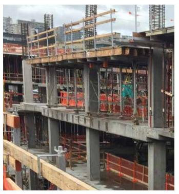
Because the SAPS guardrail system can be mounted inboard of the perimeter shoring towers, workers need to set the guardrails only once, prior to releasing and flying the exterior forms and towers to the next level. Workers outboard of the SAPS system have ready access to secure and regularly spaced tie-off points
