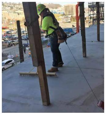
Each guardrail post provides a D-ring tie-off and brackets that clamp dimension lumber railing in place
